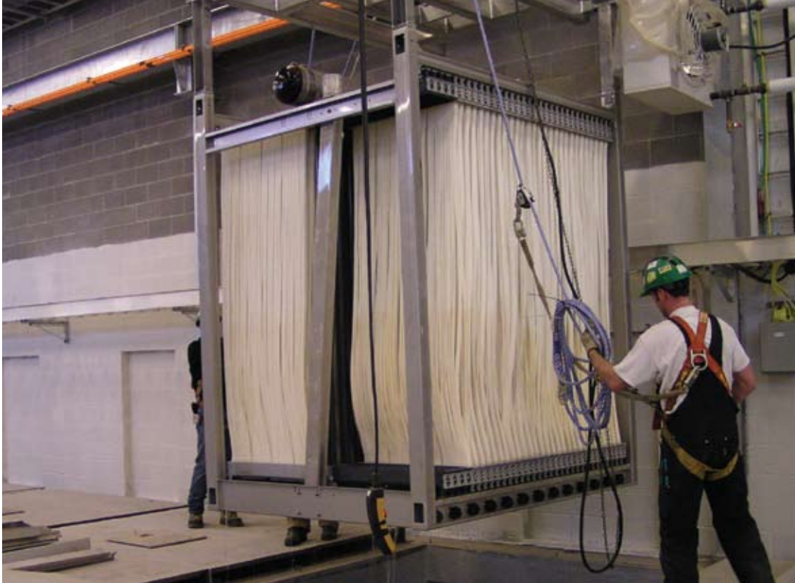
Figure 2: Membrane-based separation technology allows an increase in treatment performance and a much smaller footprint.
